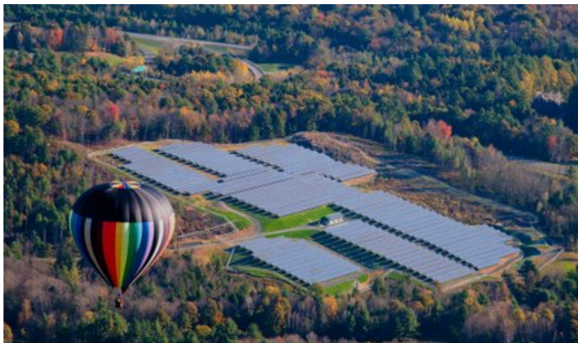
White River Junction Solar – 2.2 MW
